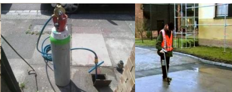
Helium Leak Detection
